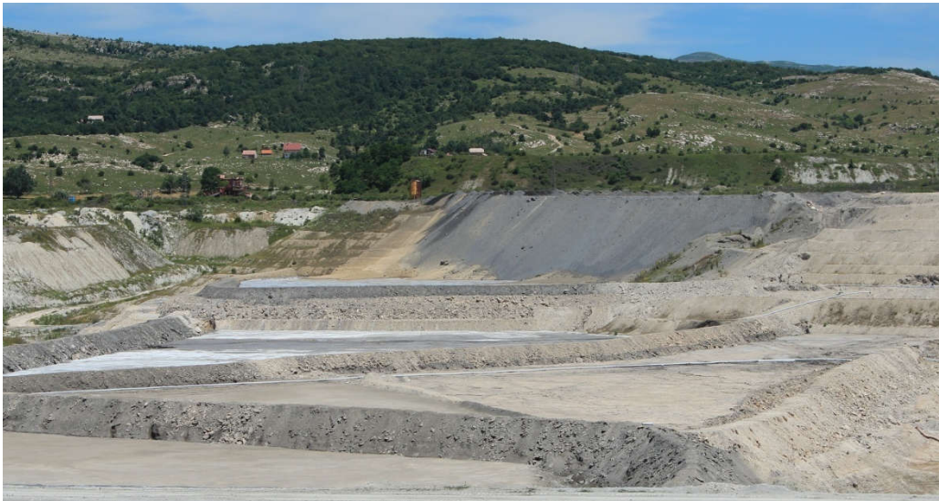
Picture 2. Internal disposal site of electrofilter ash (Cassette I i II)
