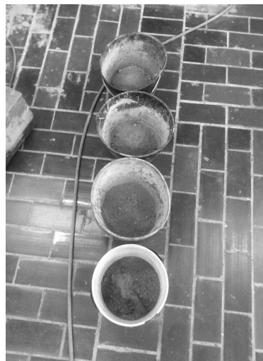
Figure 3. Preparation of earth for mud mortar
