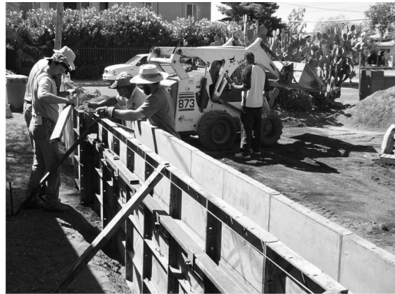
Figure 5. Placing and ramming in wall forms
