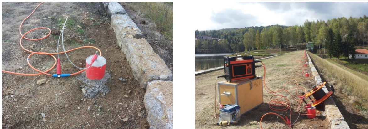
Figure 5. Fixed electrodes on the crown of the filled Vlasina dam for periodic geophysical monitoring (Vasić, 2018) [10].
