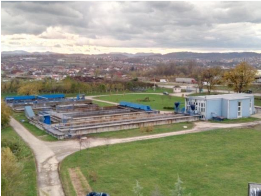
Figure 1. Wastewater treatment plant in the city of Valjevo
