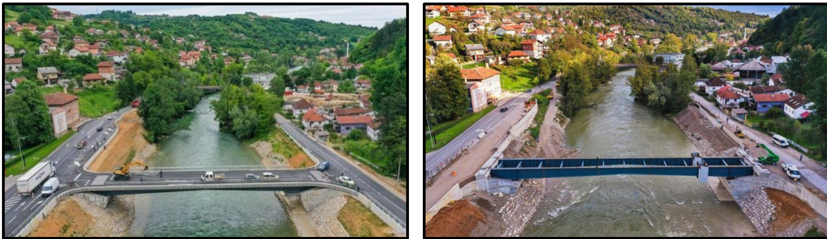
Figure 1. Road bridge over the Vrbas river, Banjaluka
