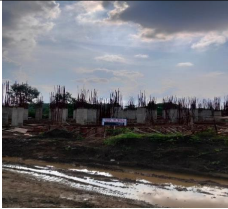
Figure 3. Construction of Duplexes
