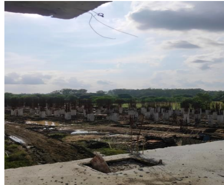
Figure 6. Top view of site under construction (SGS)
