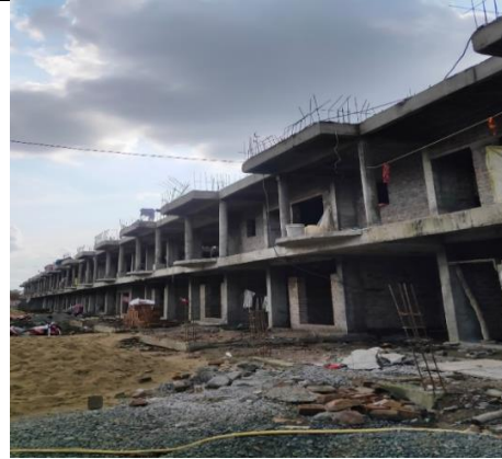
Figure 4. Ready Bungalows in campus in progress
