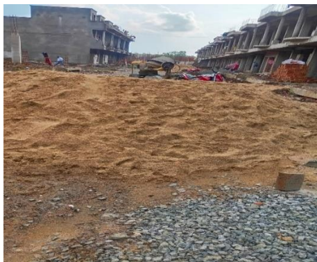
Figure 5. Post construction phase
