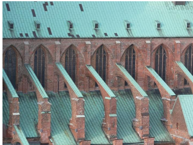
Figure 3. Arching above a side aisle roof, flying buttresses support the main vault of St. Mary's Church, in Lübeck, Germany
