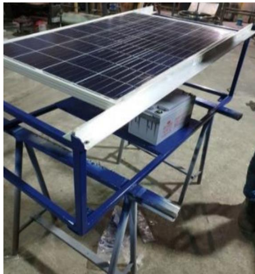
Figure 4. Fitting the Solar panel on Board
