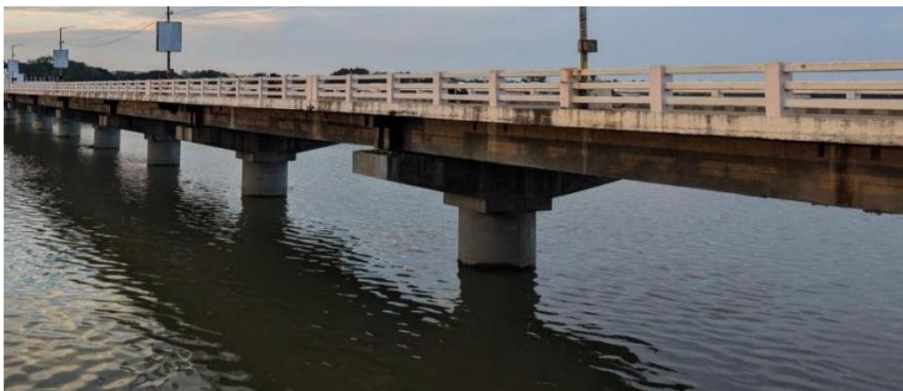
Figure 2. Swarnamukhi River Bridge, Srikalahasti, Andhra Pradesh, India
