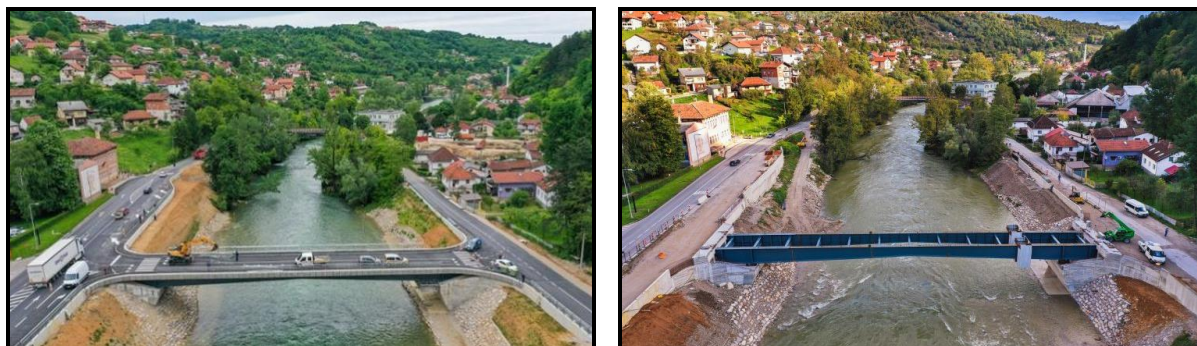
Figure 1. Road bridge over the Vrbas river, Banjaluka
